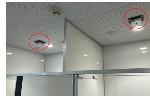
Examples of improved accessibility (Light alarm installation)
